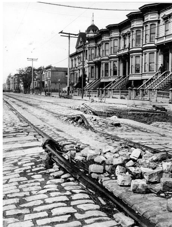
Damaged streetcar rails and cobblestone street after the San Francisco earthquake of 1906
