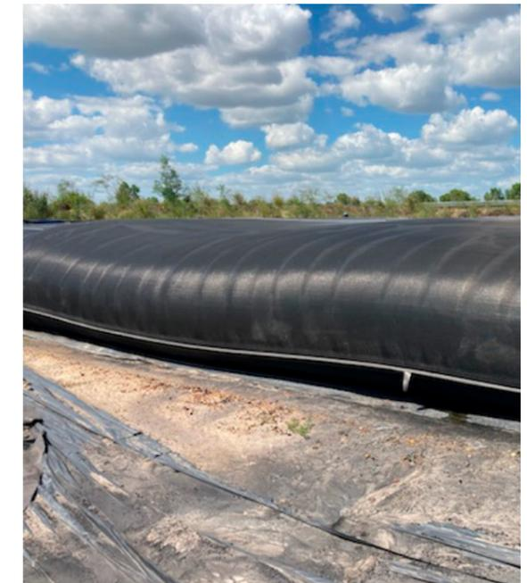
Containers are deployed on site within an available footprint to capture and dewater sludge in a confined footprint compared to open-air drying. Exposing dried coal to weather in drying beds could lead to less control over the spoil and an increased risk of re-saturation during rainfall events.
