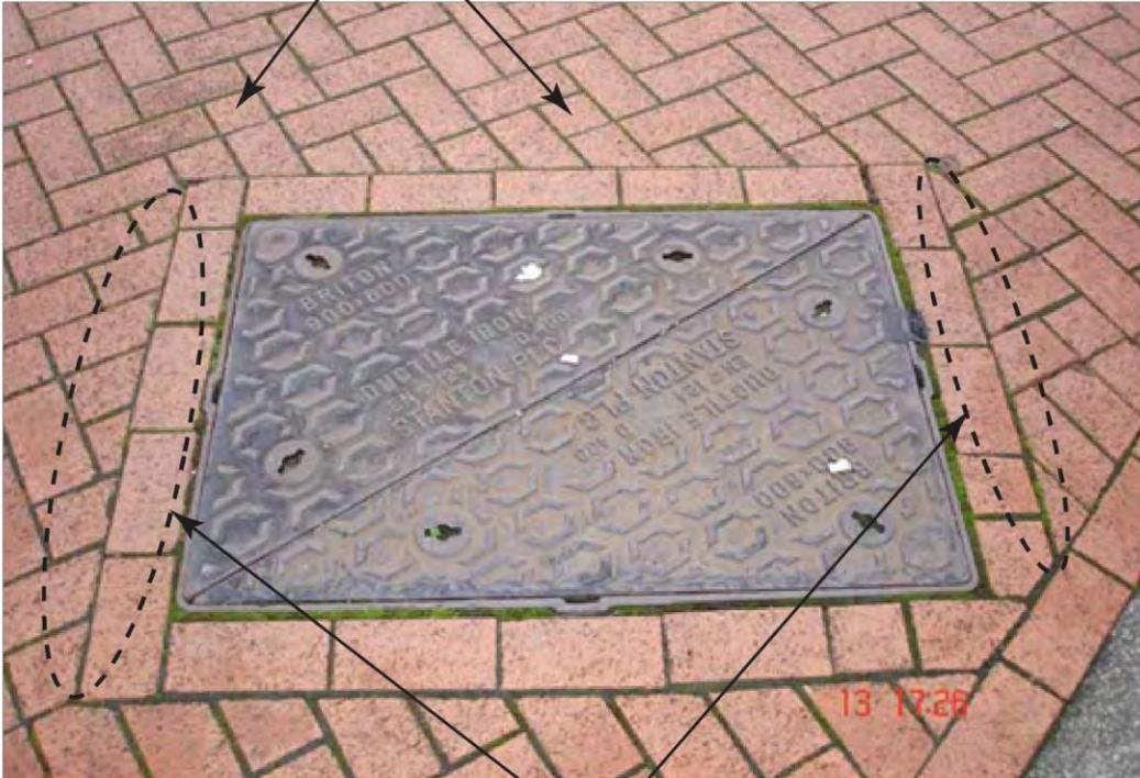
Use of larger blocks here creates acceptable loss of module pattern. This is preferred over using small angular blocks to maintain the pattern.
