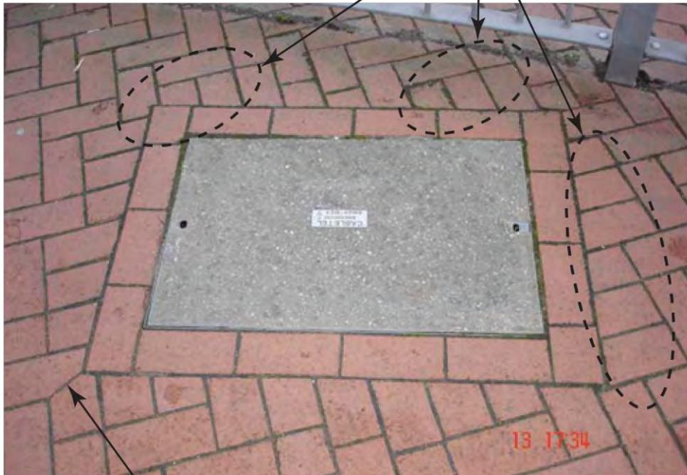
Use of larger cut blocks here leads to preferable arrangement of block pavers at the corners
