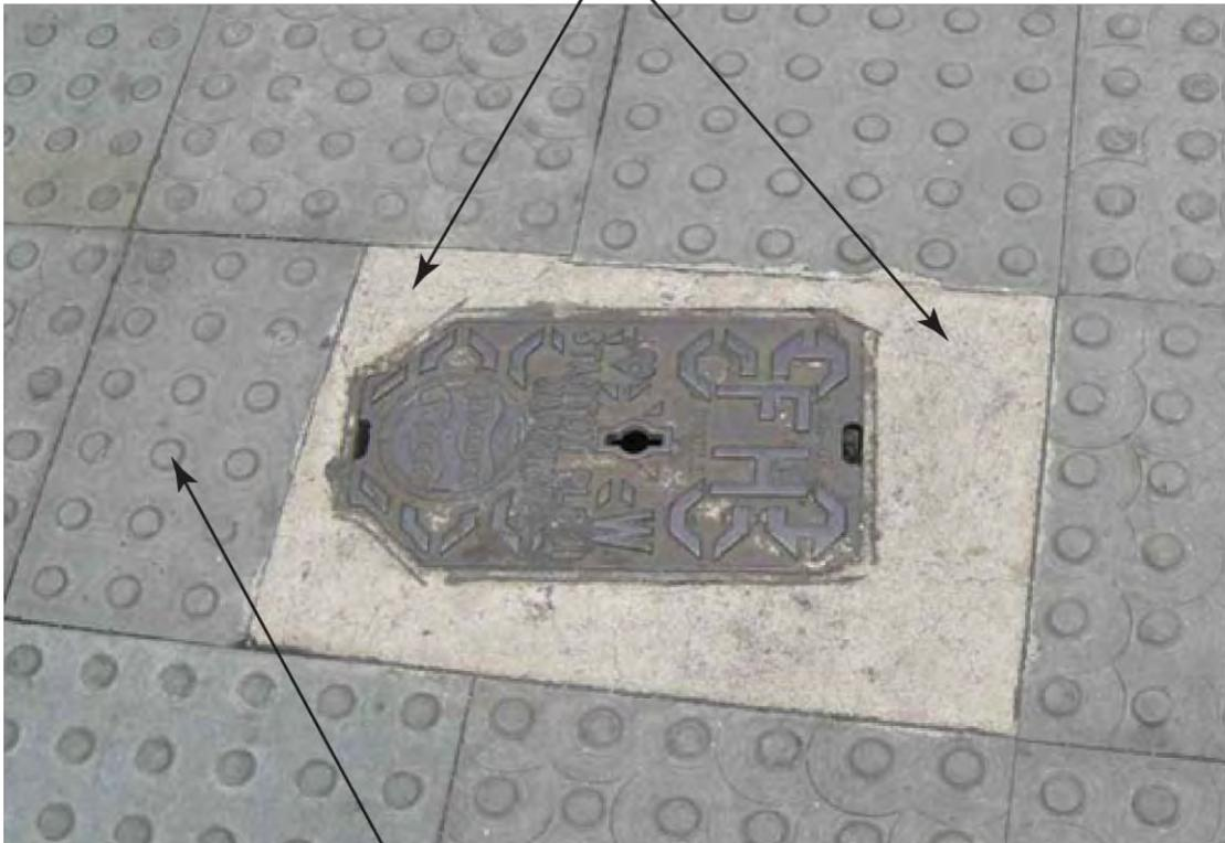
Using varying width infill limits cutting or trimming of modules
