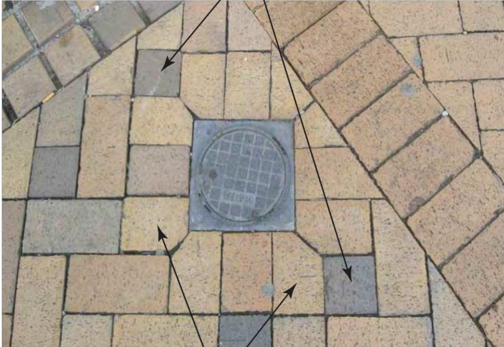
Use of larger cut blocks here creates acceptable loss of module pattern. This is preferred over using small angular blocks to maintain the pattern.
